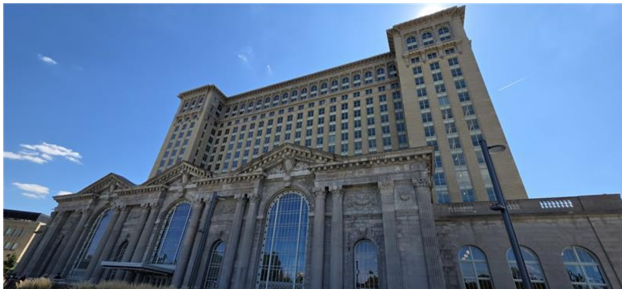
Figure 1. View on Central Michigan Station from below.
