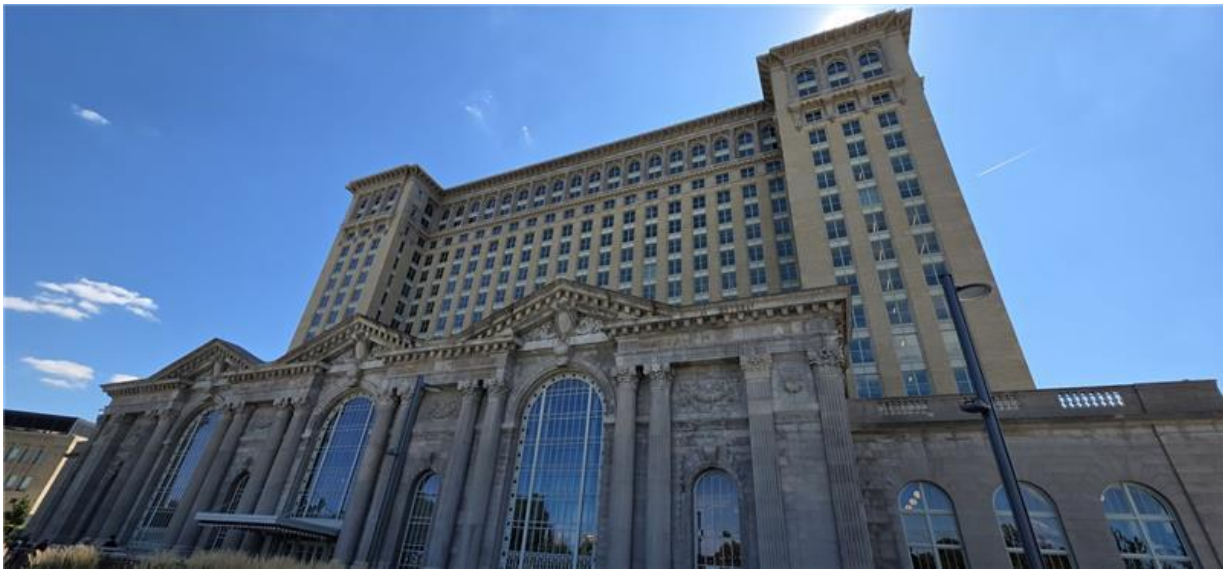
Figure 1. View on Central Michigan Station from below.
