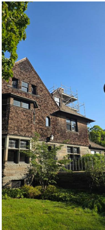
Figure 2. A view of the Freer House undergoing rehabilitation
