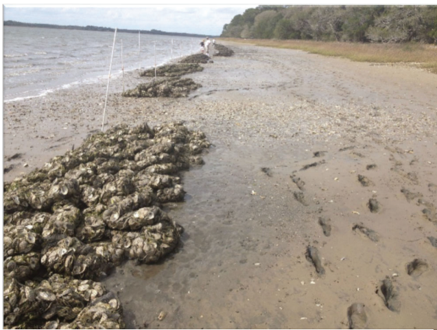
Figure 6a. The newly constructed oyster reefs at the study site in 2012. The 28 reefs are made of net bags of recycled oyster shells.
