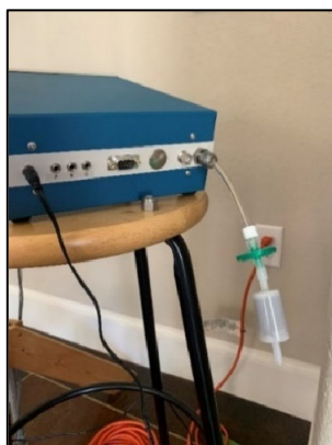
Figure 2A. Ozone scrubber attached to ozone monitor.
